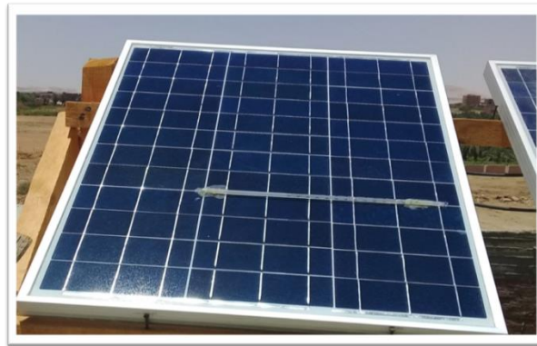
Figure (3): The polycrystalline photovoltaic module is angled 30 degrees southward to face the sun
