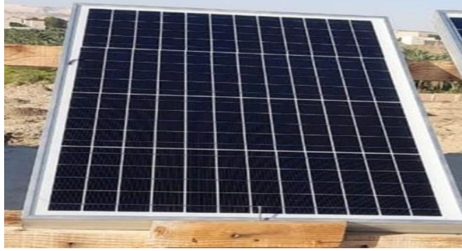
Figure (2): The monocrystalline photovoltaic module is angled 30 degrees southward to face the sun.
